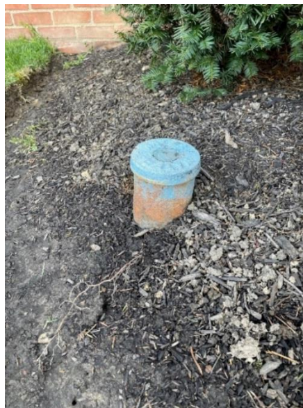
Master water cap sticking up about 4-5"
