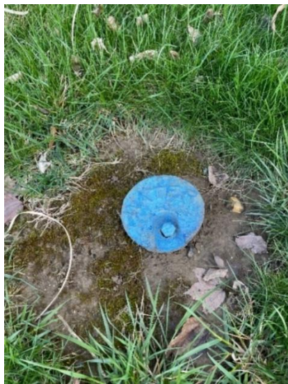
Master water cap flush to ground
